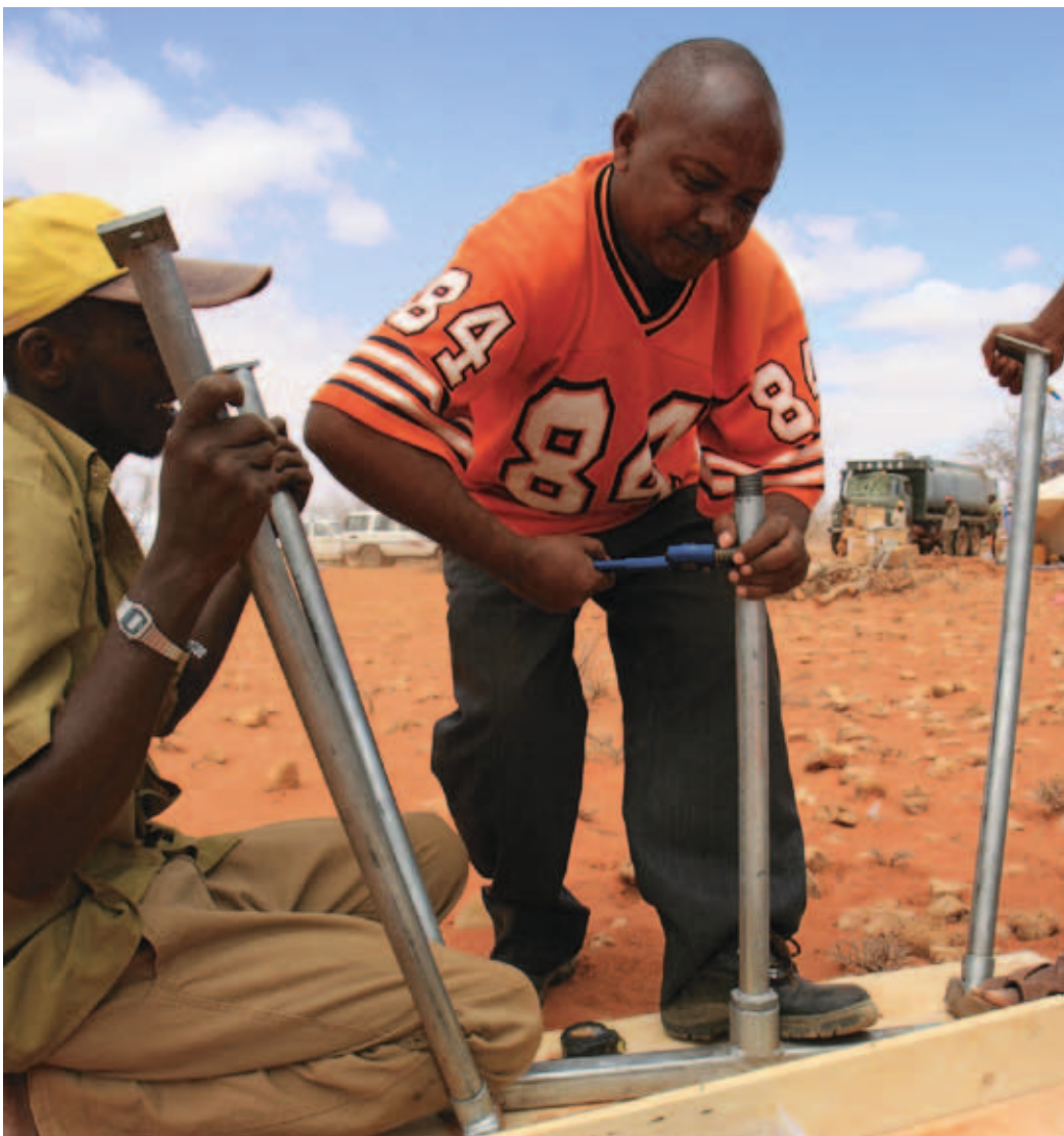
◀ Abbra, an Oxfam driver, lends his efforts to helping make the camp ready for the refugees by assembling tapstands sent from the UK. Photo: Jane Beesley.
